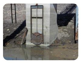
4. Once drain is closed and if visible, attempt to inspect and ensure there is no debris or build-up that could hinder flow.
