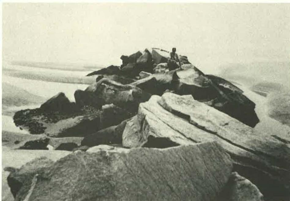
Figure G-10. The jetty located on the south end of Cumberland Island is acting as a sediment trap causing growth of the island.
