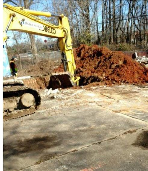
Photo of over excavation in progress.
