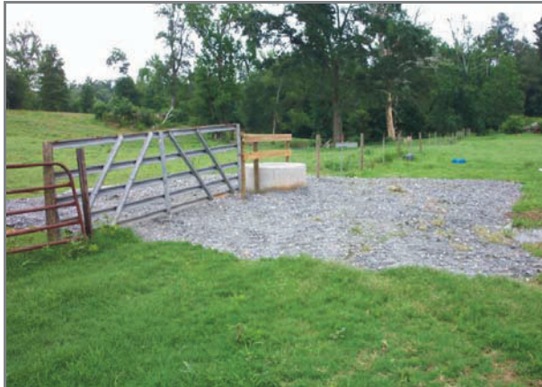
Heavy Use Area Protection around a watering trough
