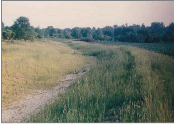
A grassed diversion is planted to redirect water from a slope and also traps nutrients and sediment in runoff
