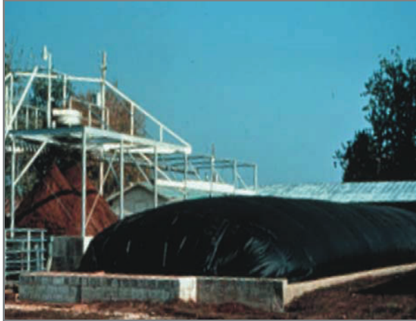
An operational anaerobic digester
