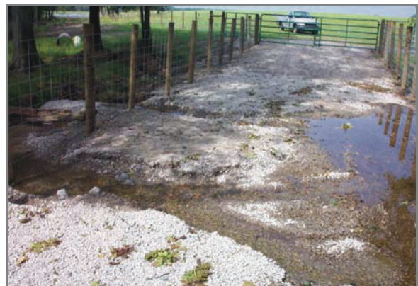
A ford installed as a stream crossing
