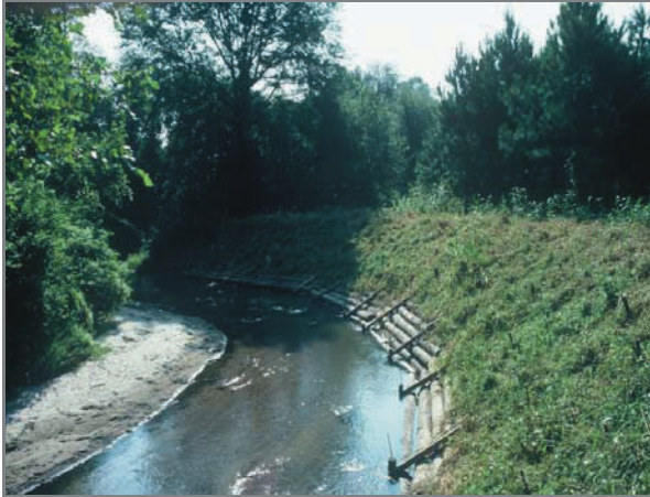
A stream revetment was used to reduce and prevent streambank erosion along with revegetation
