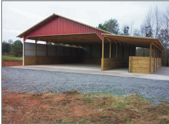
A stack house allows for litter storage until it can be used for other purposes or can be transported off-farm
