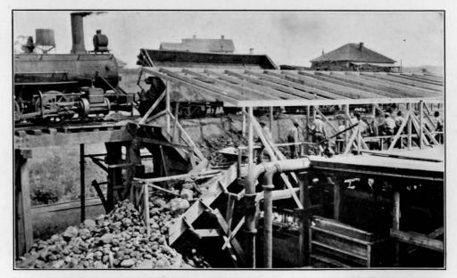
B VIEW SHOWING MANGANESE ORE BEING DUMPED ONTO THE GRIZZLIES AT THE AUBREY PLANT OF THE GEORGIA IRON & COAL COMPANY, WHITE, BARTOW COUNTY.
