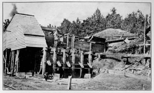
A. CONCENTRATING MILL SHOWING ARRANGEMENT OF LOG WASHER, SCREEN, AND JIGS AT THE STILES MINE, ETOWAH DEVELOPMENT COMPANY PROPERTY, 2 MILES EAST OF CARTERSVILLE, BARTOW COUNTY.
