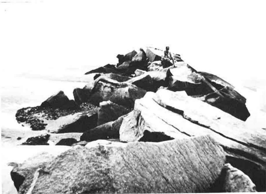
Figure 18. Jetty located on the south end of Cumberland Island. Because the jetty acts as a sediment trap, the island has enlarged considerably updrift of this location.
