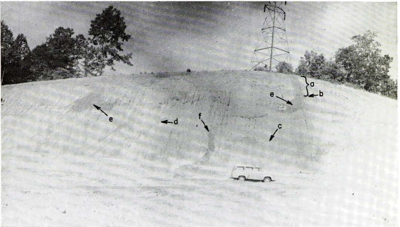
Figure 9.—Seeps show paths of water movement in saprolite. Road cut is near Doraville, DeKalb County. (See p. 20 for explanation.)
