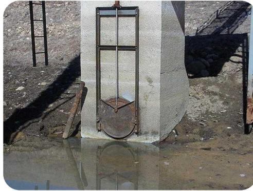
4. Once drain is closed and if visible, attempt to inspect and ensure there is no debris or build-up that could hinder flow.
