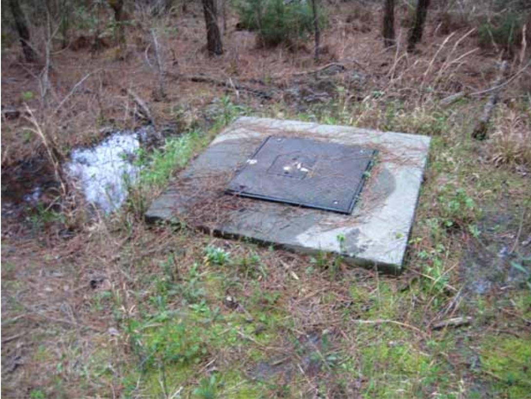
**Photograph No. 20:** Water inside RW-4 cover from probable leaking recovery pump line.
